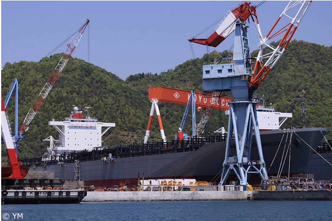
K-Line's new SAN DIEGO BRIDGE is seen here under construction at Imabari's Koyo Dockyard at Mihara, Japan. Several weeks...
