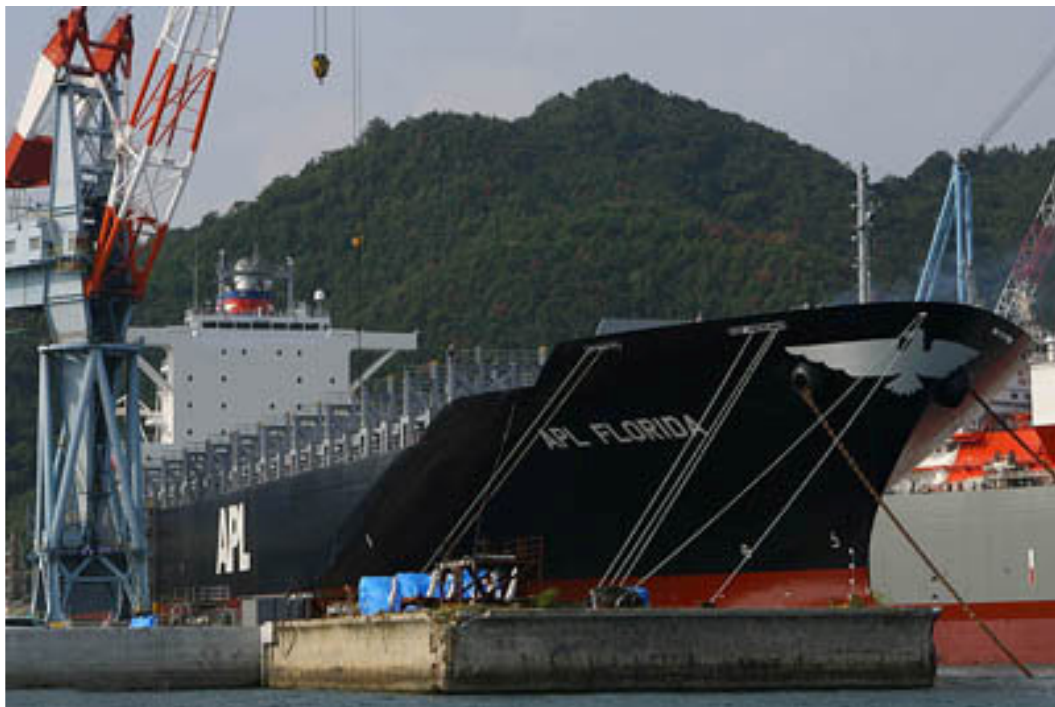
This shot, taken at Mihara, shows the Koyo-built 6,350 teu container vessel APL FLORIDA nearing completion... photographer: Y.M. (anonymus)
