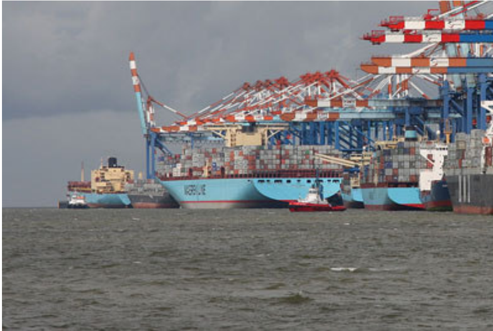
Terminal VI at the northern end of Bremerhaven's Stromkaje is clearly in the hands of Maersk Line.
